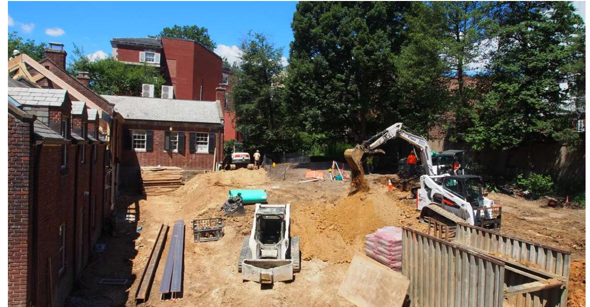
In the upper left, carpenters continue to frame the new roof over the Carriage House deck. On the right, excavators dig a trench for an 8-inch drain line that will serve drains on the upper terrace.
