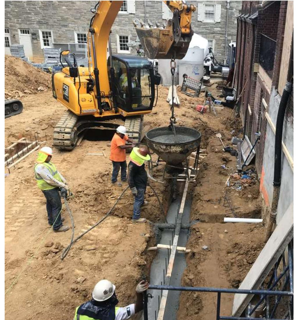
The pipe running across the footing is a new drain pipe from the soon-to-be-renovated Quaker House Boiler Room.
