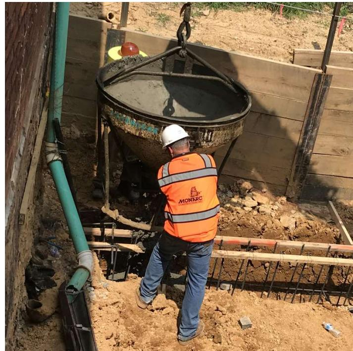
The wall that will rest on this foundation will hold back the dirt of the upper terrace on the right and will form the north wall of the new Storage Room on the left.
