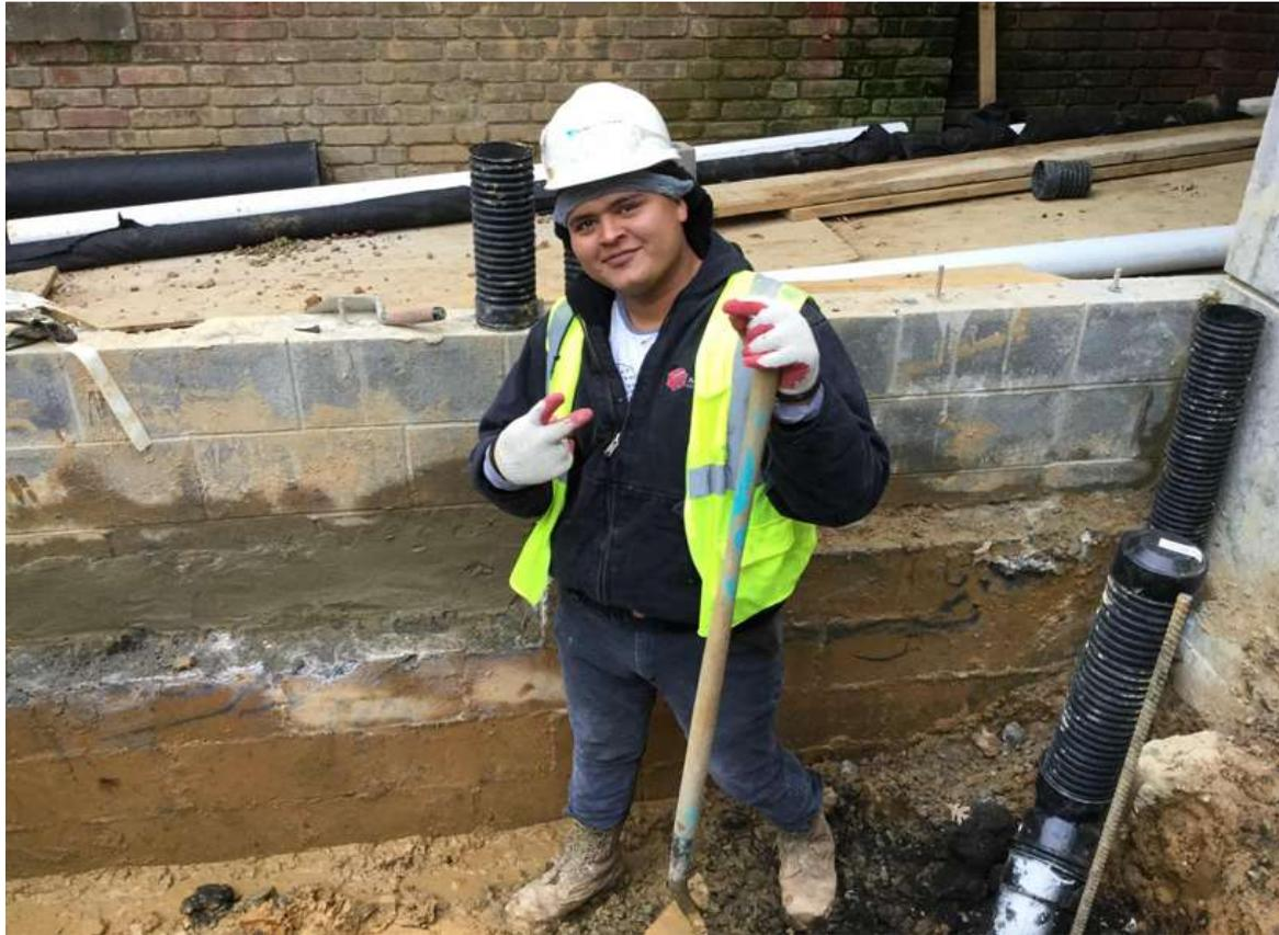
He's engaged in helping to clean the mud off the foundation so that parging (a thin protective layer of concrete) can be applied.
