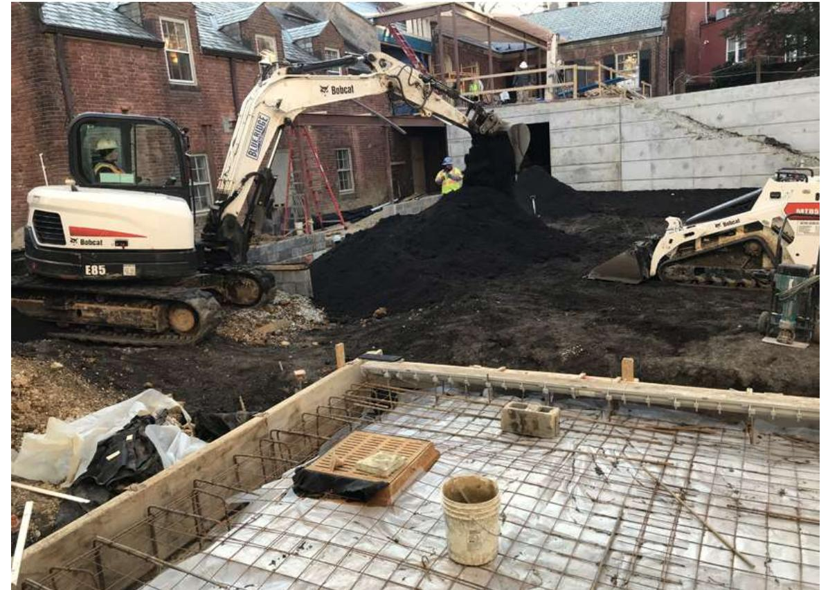
while steel mesh is installed around the drains to reinforce the new patio.
