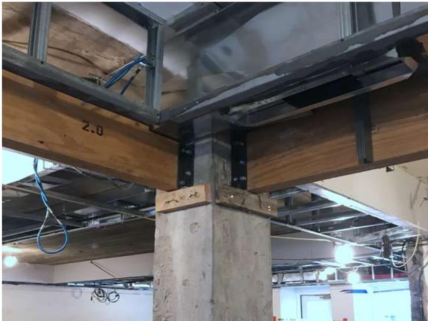
LVL (laminated veneer lumber) is engineered wood, like plywood, but with the wood grain all running along the beam, like real timber, only stronger and more stable.
