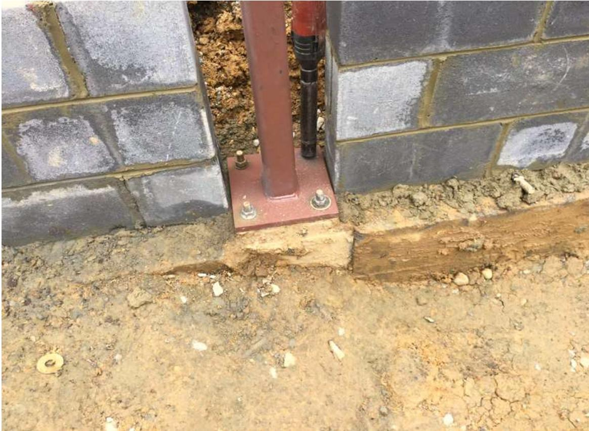
This post, being bolted to the corridor foundation, will be cemented into the adjoining stem walls and support the Carriage House upper corridor and roof.
