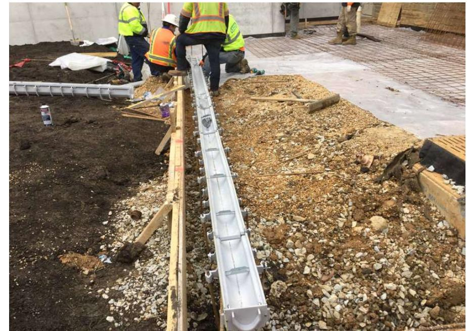
They also install the last drainage connection to tie new downspouts into the new drainage system.
