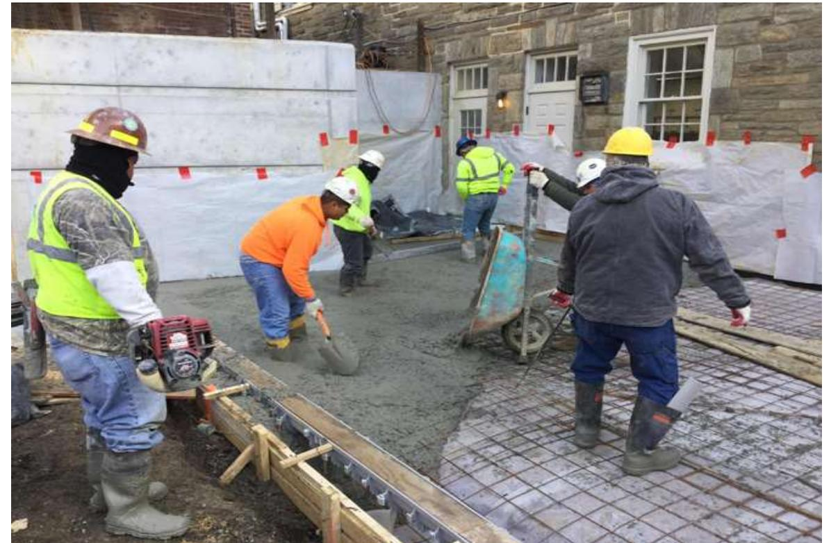
It's going to be a cold night, and concrete should stay above 40° when it's setting, so they cover it with a blanket.
