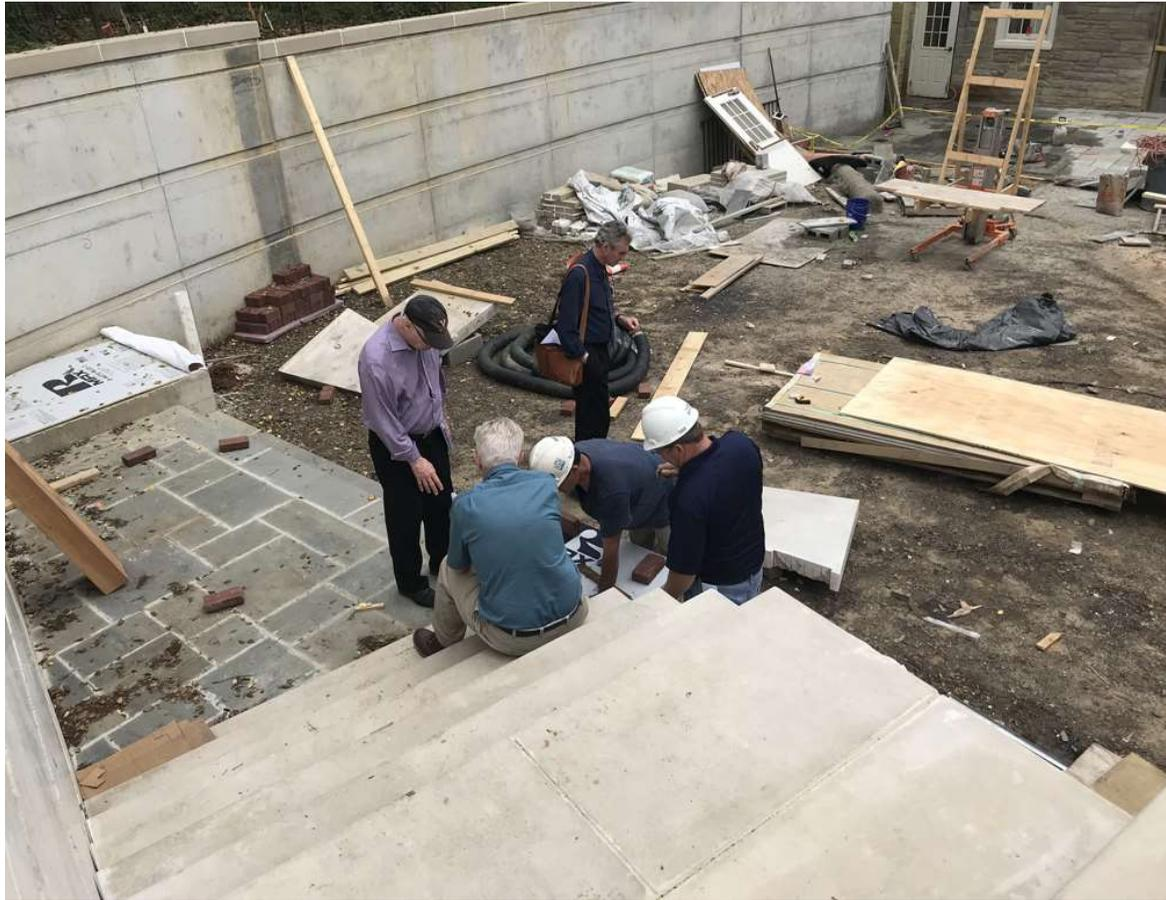
The big chunks of cast stone on the ground are capstones that were installed, judged not quite right, and taken off again.
