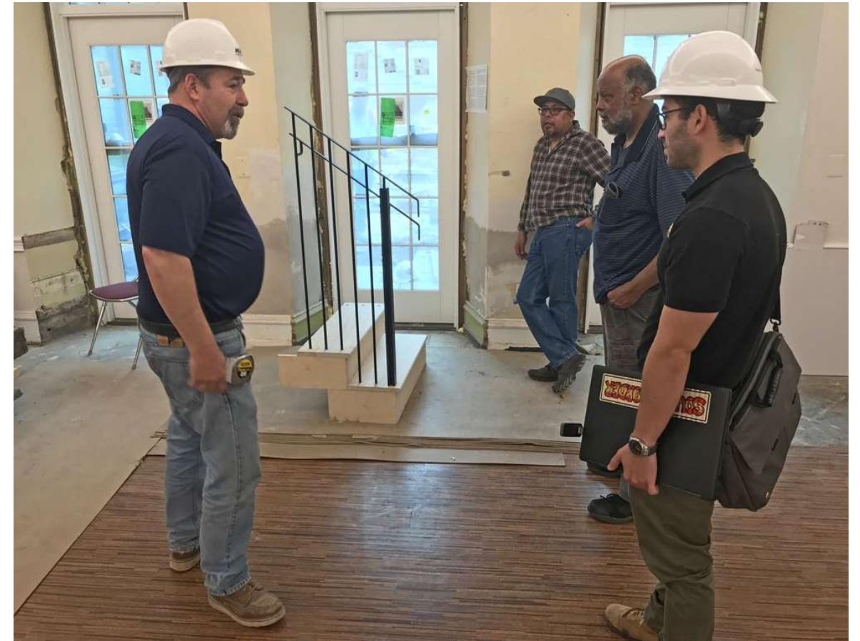
This is a mockup of the planned Lobby stairs, created by the ironworkers and carpenters, so the architects can approve the details before construction.
