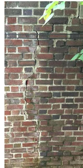
A crack has appeared in the Embassy wall, probably caused by the combination of nearby excavation and rain.
