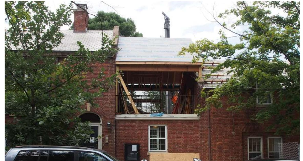
They also install roof jacks (just to the right of the roof in the above picture) to support a platform so they can temporarily relocate the heat pump compressor (now on the deck) to provide continued service to Carriage House during the work.
