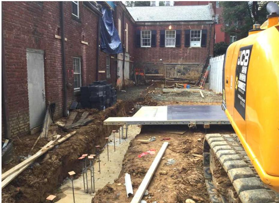
Then they install the reinforcing steel and frame out a void for the double doors that will open out into the Assembly Room Terrace.
