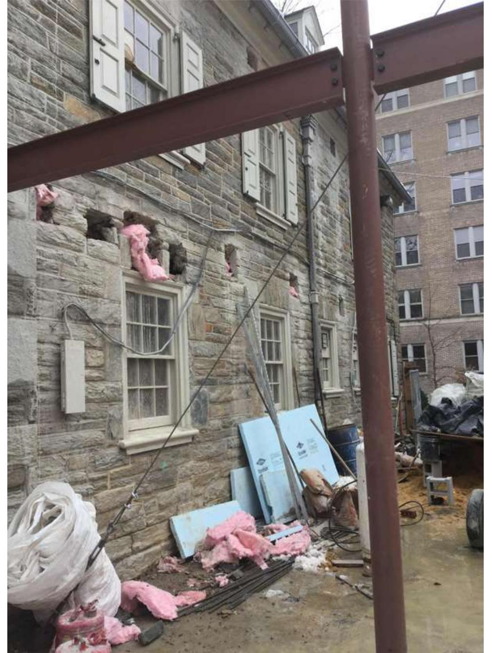
The masons dig right in, opening up the wall even more to build up the new lintel on this side.
