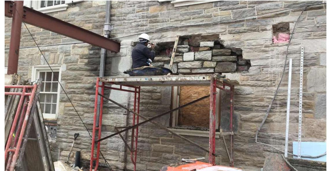
On the other hand, they are sawing through the wall below the Assembly Room doors and windows and chipping away at the stone.
